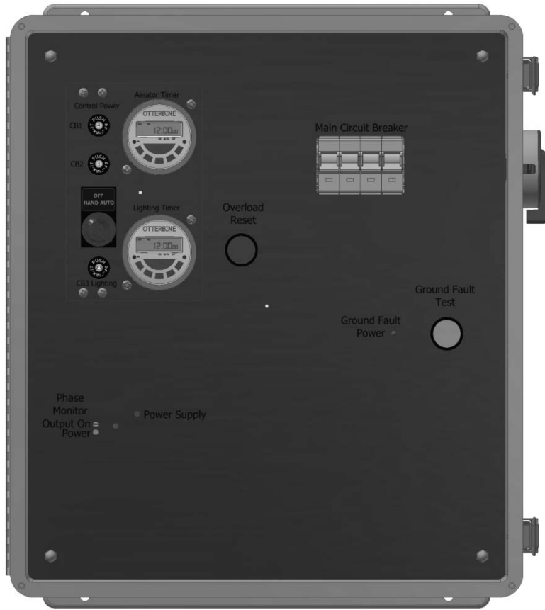
Three Phase Panel
